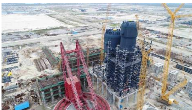
Fig. 16: World's largest Reactor-Regenerator Supporting Structure
