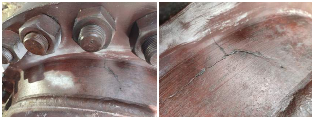
Fig.1-2: Multi-branched cracks at leakage location
