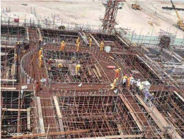
Fig. 12: Casting of Regenerator Supporting Beams
