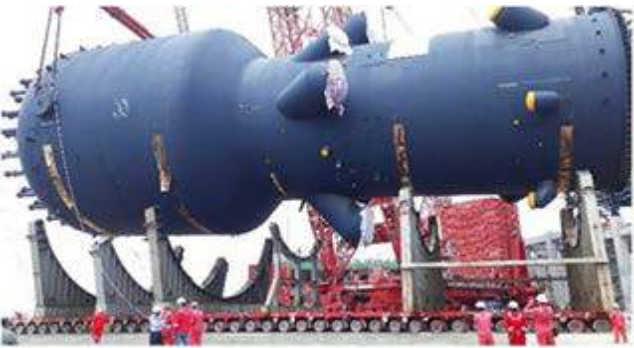
Fig. 9: Regenerator Transportation in Single Piece
