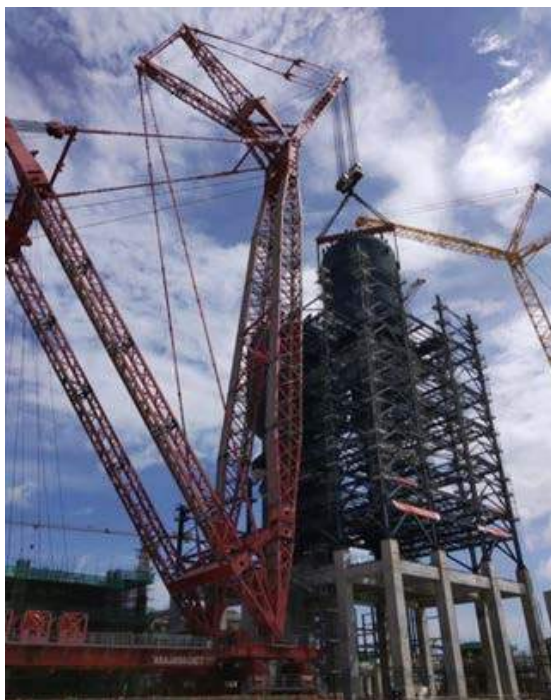
Fig. 15: Reactor Erection
