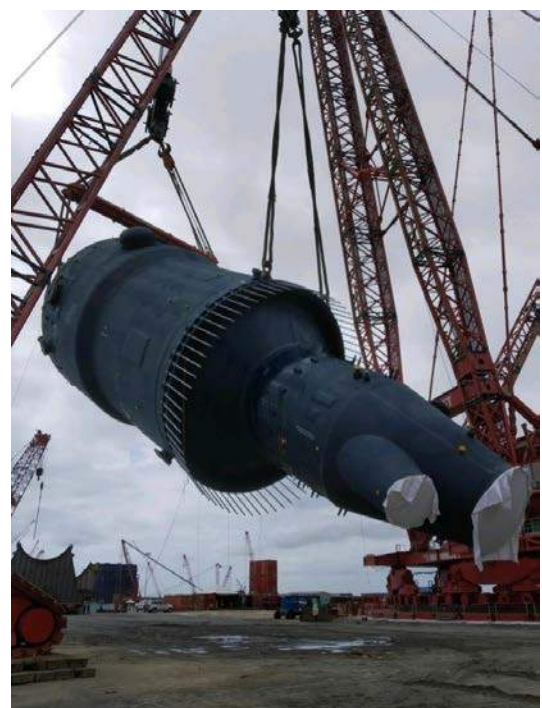
Fig. 14: Regenerator Erection
