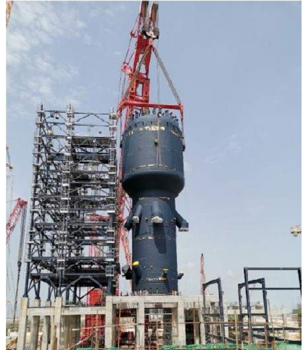
Fig. 14: Regenerator Erection
