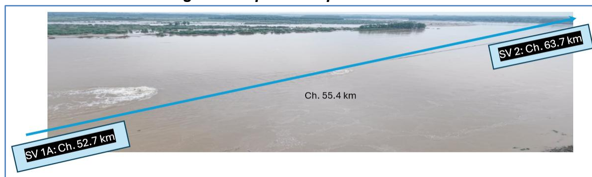
Figure 2: Pipeline Rupture Location
