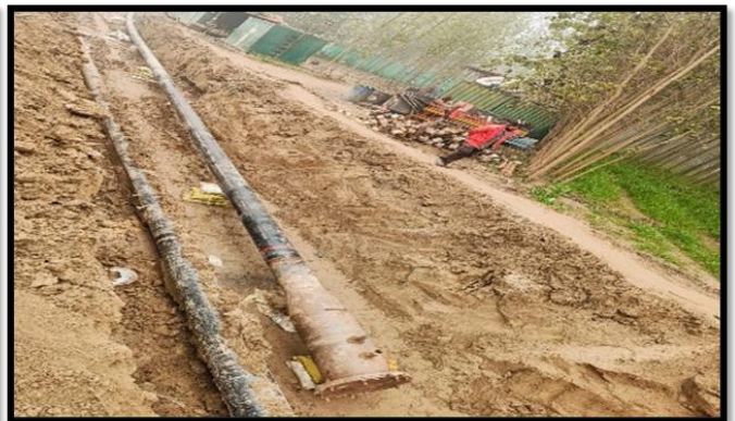
Figure 16 Hook Up with Existing Pipeline
