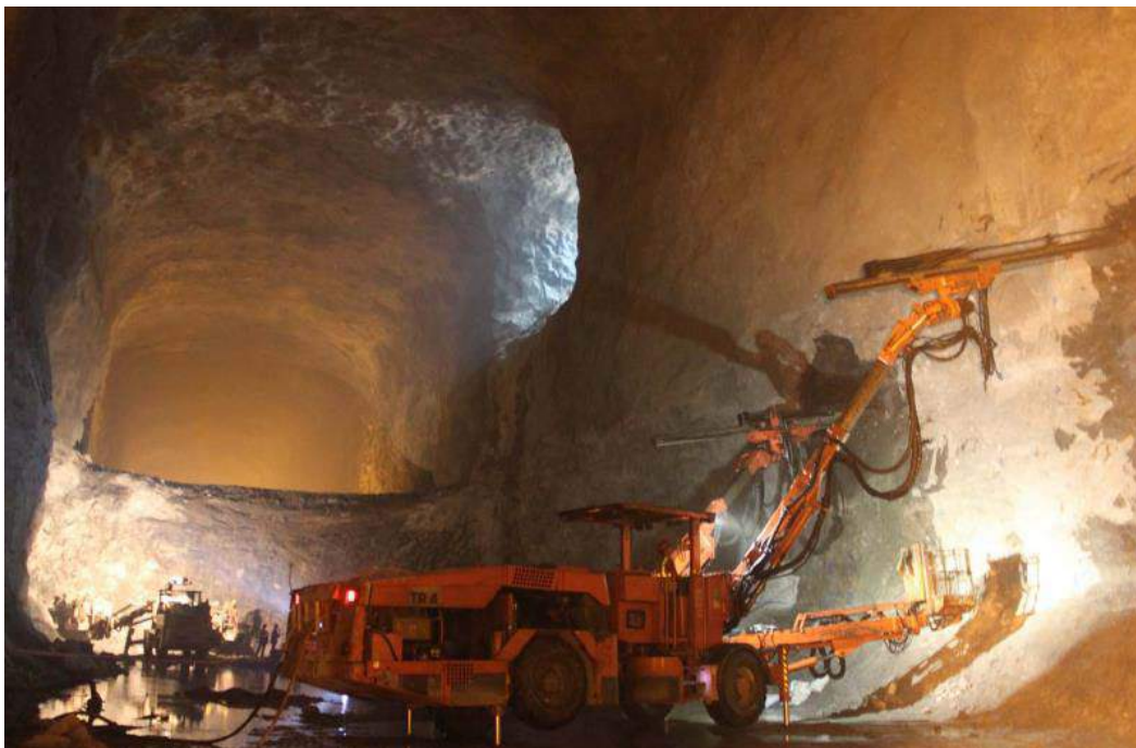
Figure 6: Cavern excavations in stages
