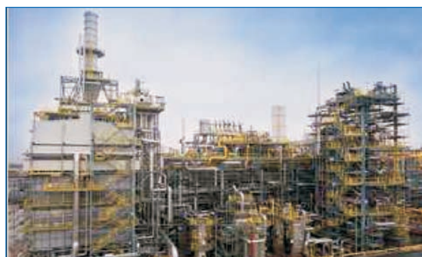
Exhibit 3: LUKOIL H-Oil Unit in Bulgaria
