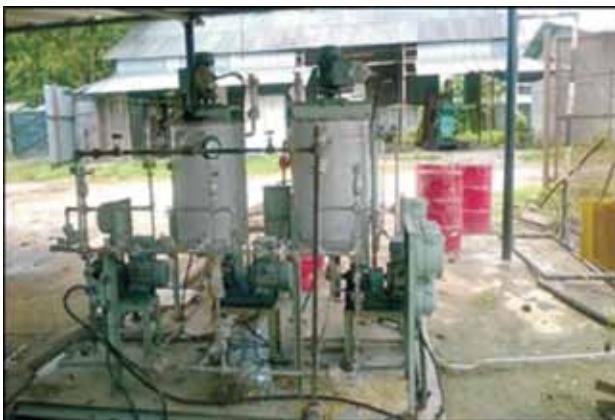
A chemical injection set-up
