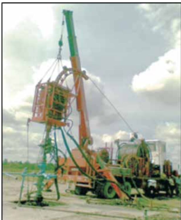
Coil Tubing Unit used for hot oil circulation in the tubing
