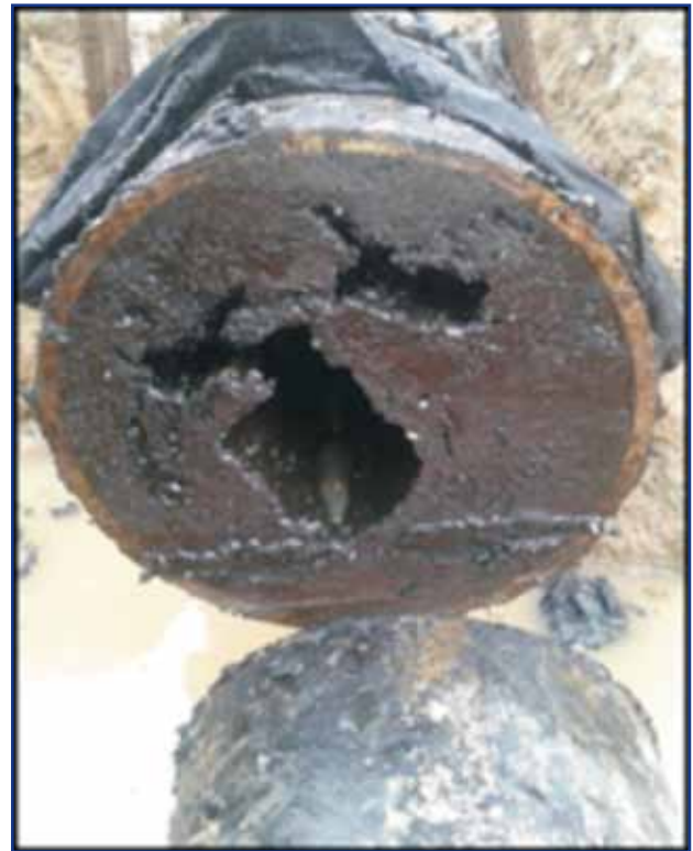
Organic deposits seen in the cross-section of a cut-out portion of a pipeline
