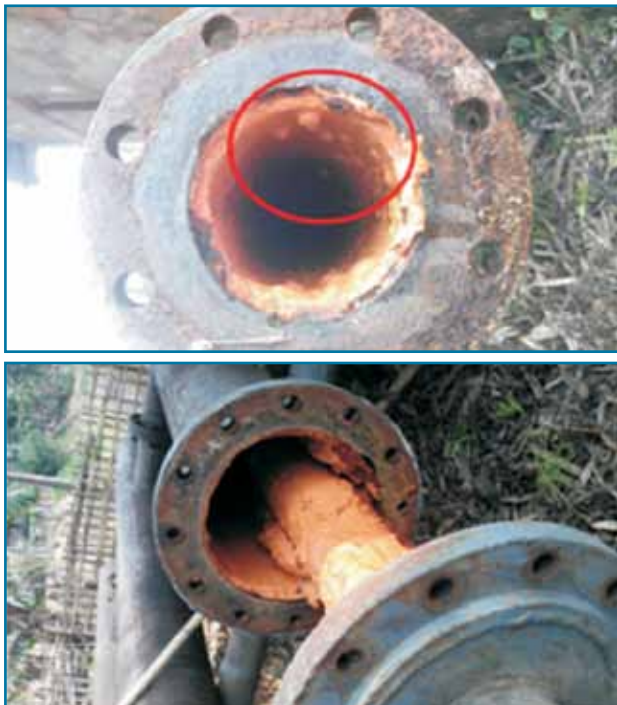
Figure 6: Microbial induced corrosion in water injection manifolds
