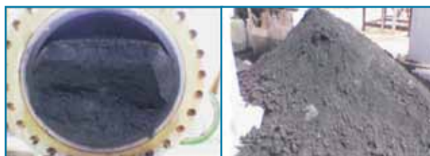
Figure 8: Black powder (Siderite) problem in Natural Gas pipelines is owing to CO_2 /Erosion corrosion
