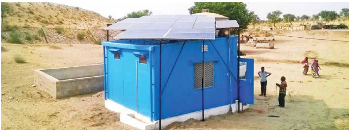
India's largest solar operated community based RO Plant has been installed at Sewniwala in Baytu Tehsil.
